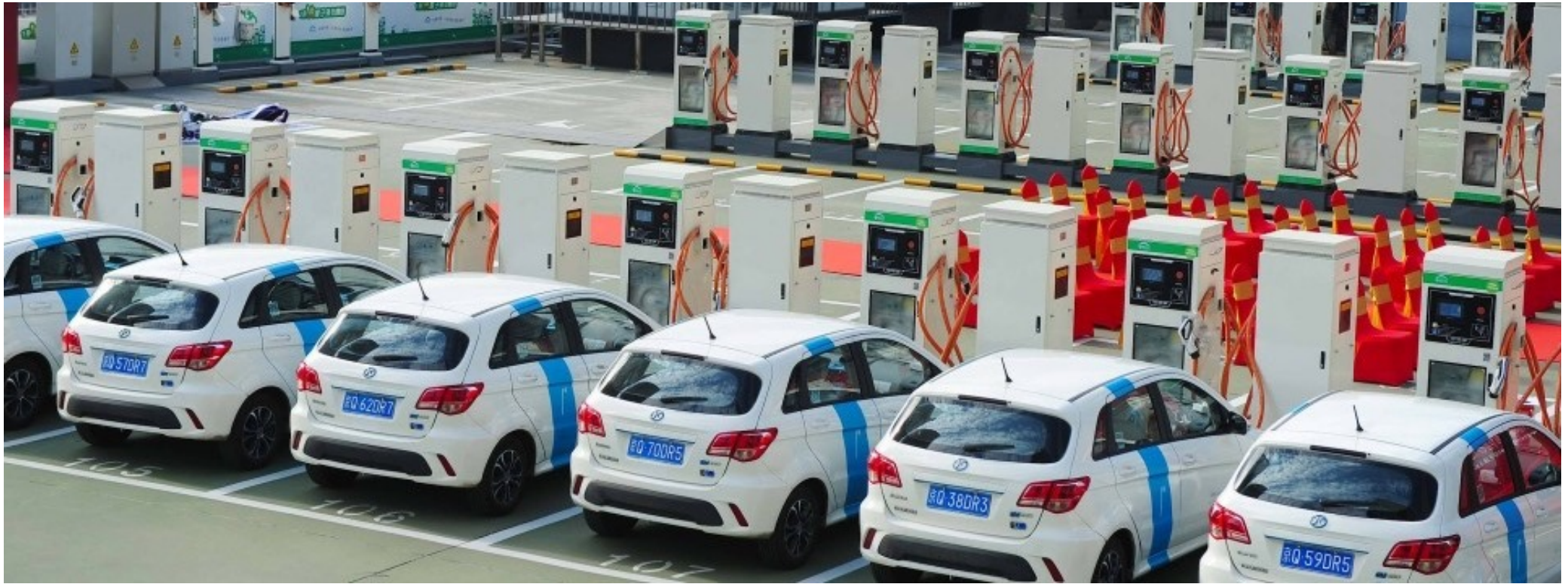
Rooftop of a parking garage Beijing
